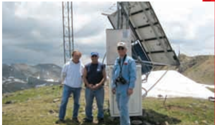
We assist in repairing a Ham repeater at 13,400 feet.
